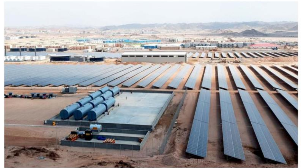
NEOM CITY - TAMIMI ENERCO PROJECT / NEOM CONSTRUCTION VILLAGE
