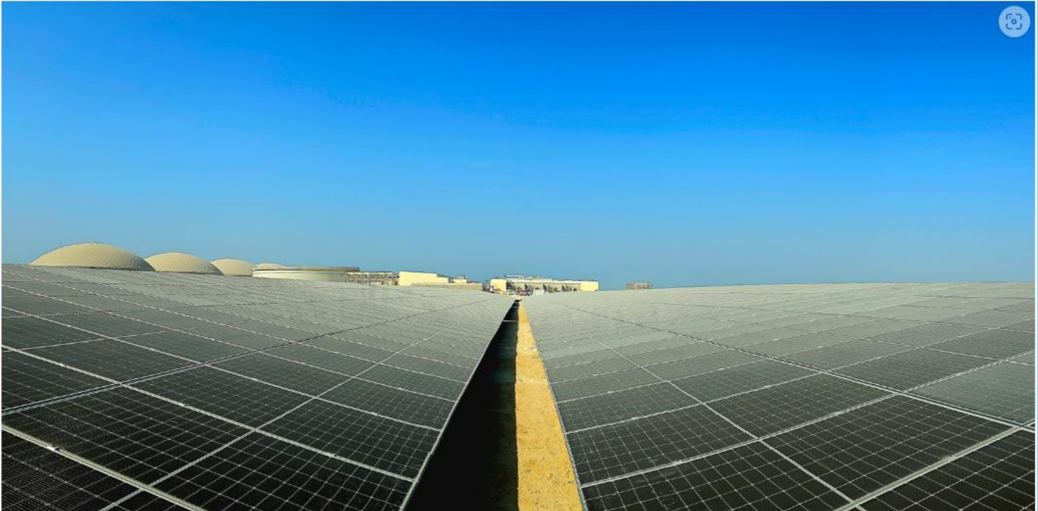
ACCIONA Project location :Saudi Arabia-Jubail Project Capacity : 65MW
